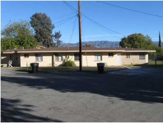
Original Unit Condition
