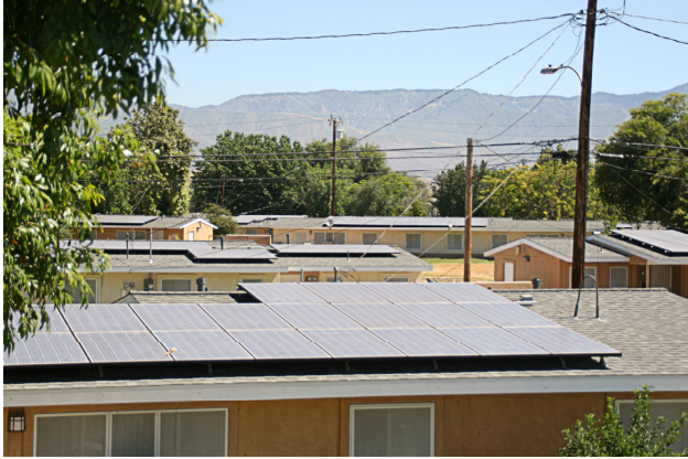
View of Rooftops with Solar Panels at Maplewood Homes
