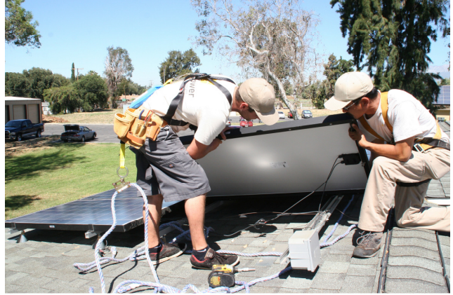
Workers Installing Solar Panels
